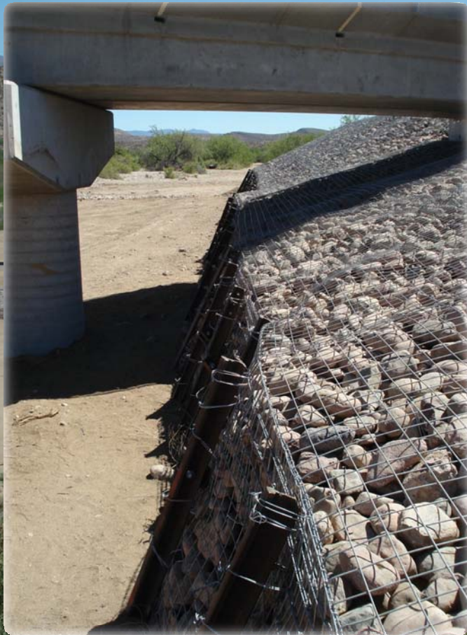
Bank protection at abutments
