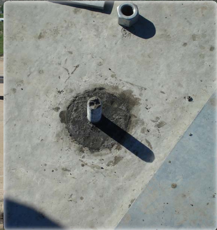
Pinned connection
