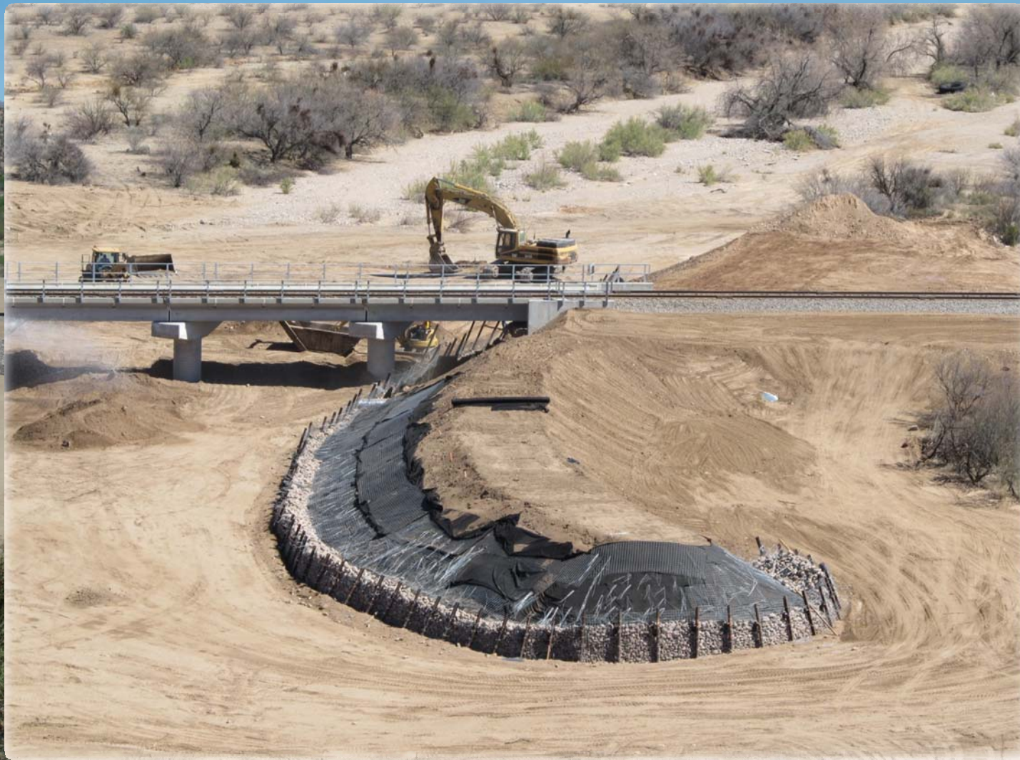
Bank protection in progress with filter fabric and rock
