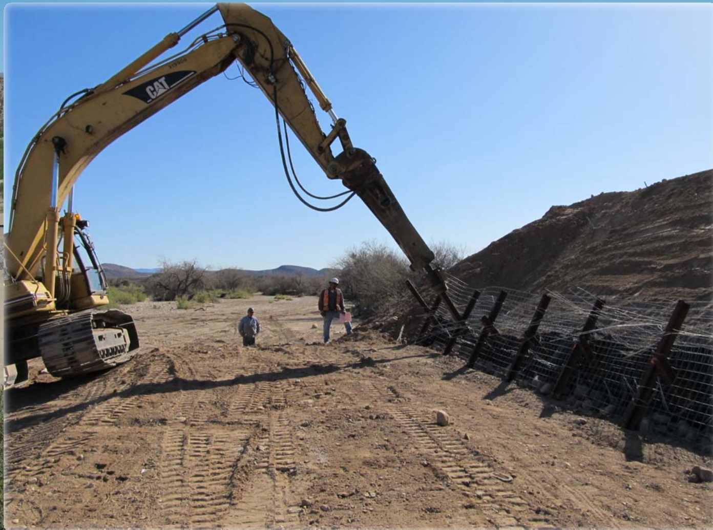
Installing short rails
