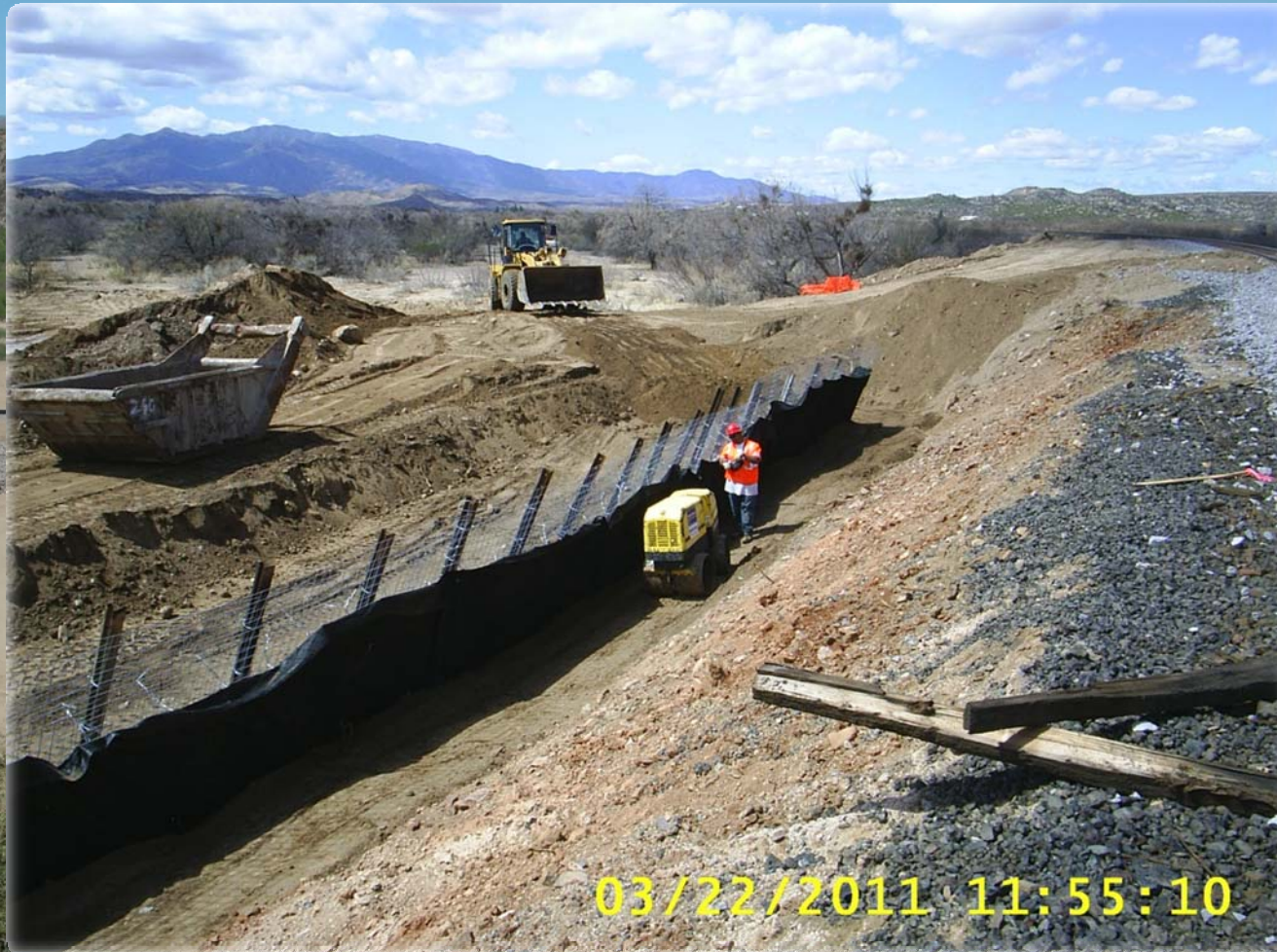
Backfilling behind bank protection with remote control compactor
