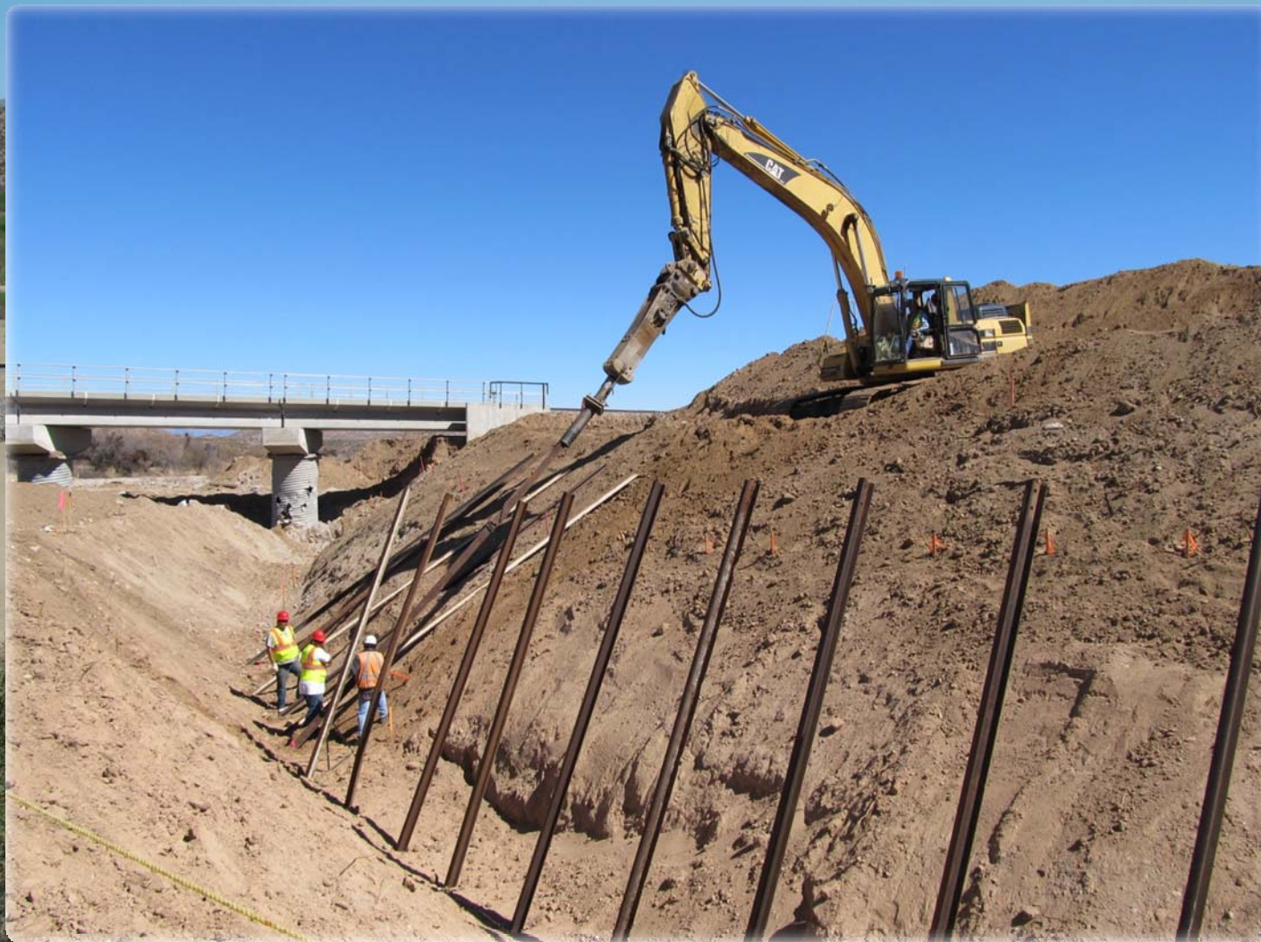
Installation of long rails on overexcavated slope (1.5H:1V)
